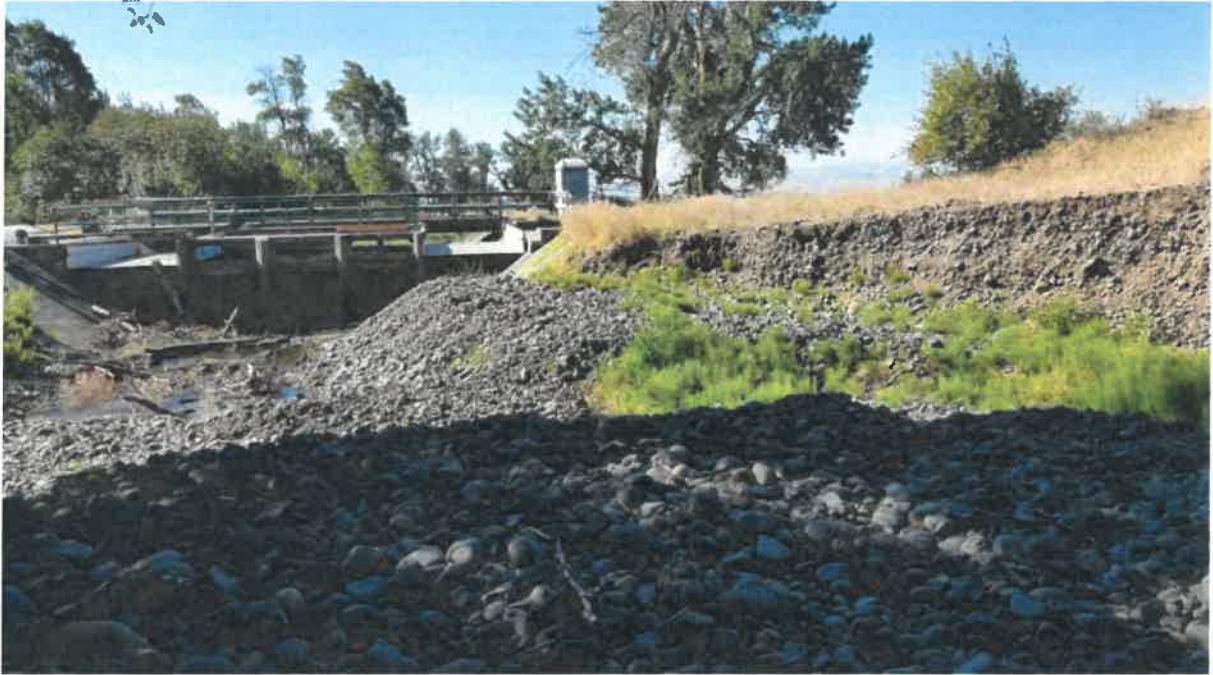
Photo 3. Eroded bank just upstream of the KRD canal intake structure that requires armoring. Sediment deposition in the channel forced the creek into this bank, causing rapid erosion.
