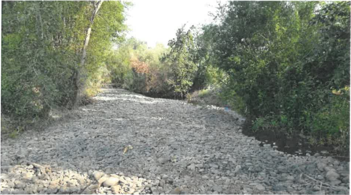
Photo 1. Accumulated sediment upstream of the KRD canal intake has forced Naneum Creek out of the current channel. Naneum Creek flows are seen on the right edge of the photo. Keeping flows isolated like this will allow a dry work area for equipment.
